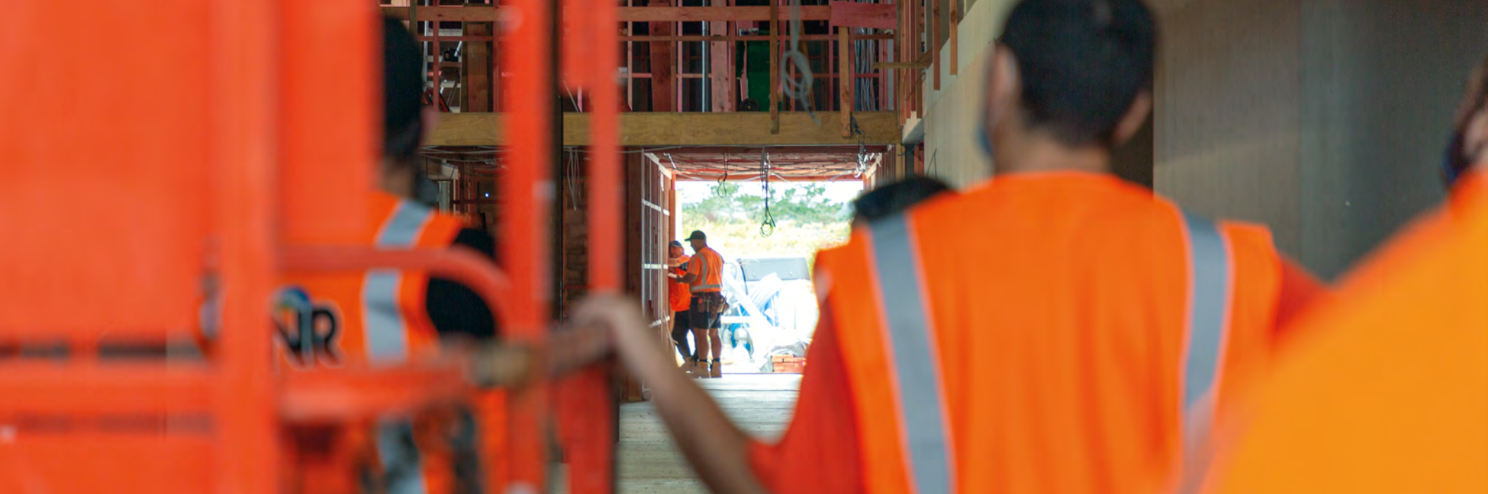
Above Construction workers at the Kā Uri site, February 2022.
